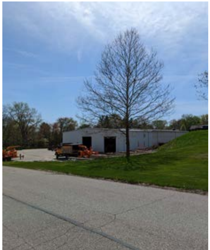
Franklin Park Borough Public Works Garage
