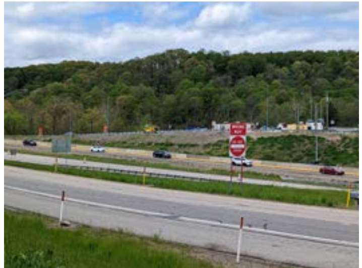
View of I-79 from the Park & Ride Lot at the Intersection of Mount Nebo Road and Red Mud Hollow Road
