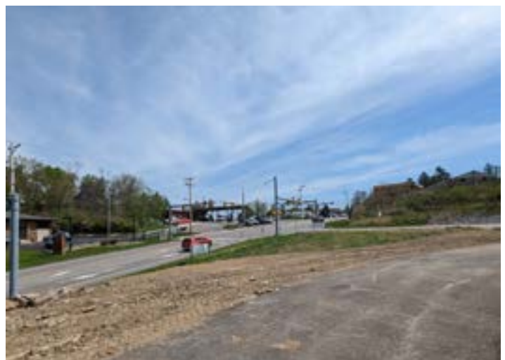
Sewickley Pointe Parcel and Pad Sites on Mount Nebo Road in Ohio Township
