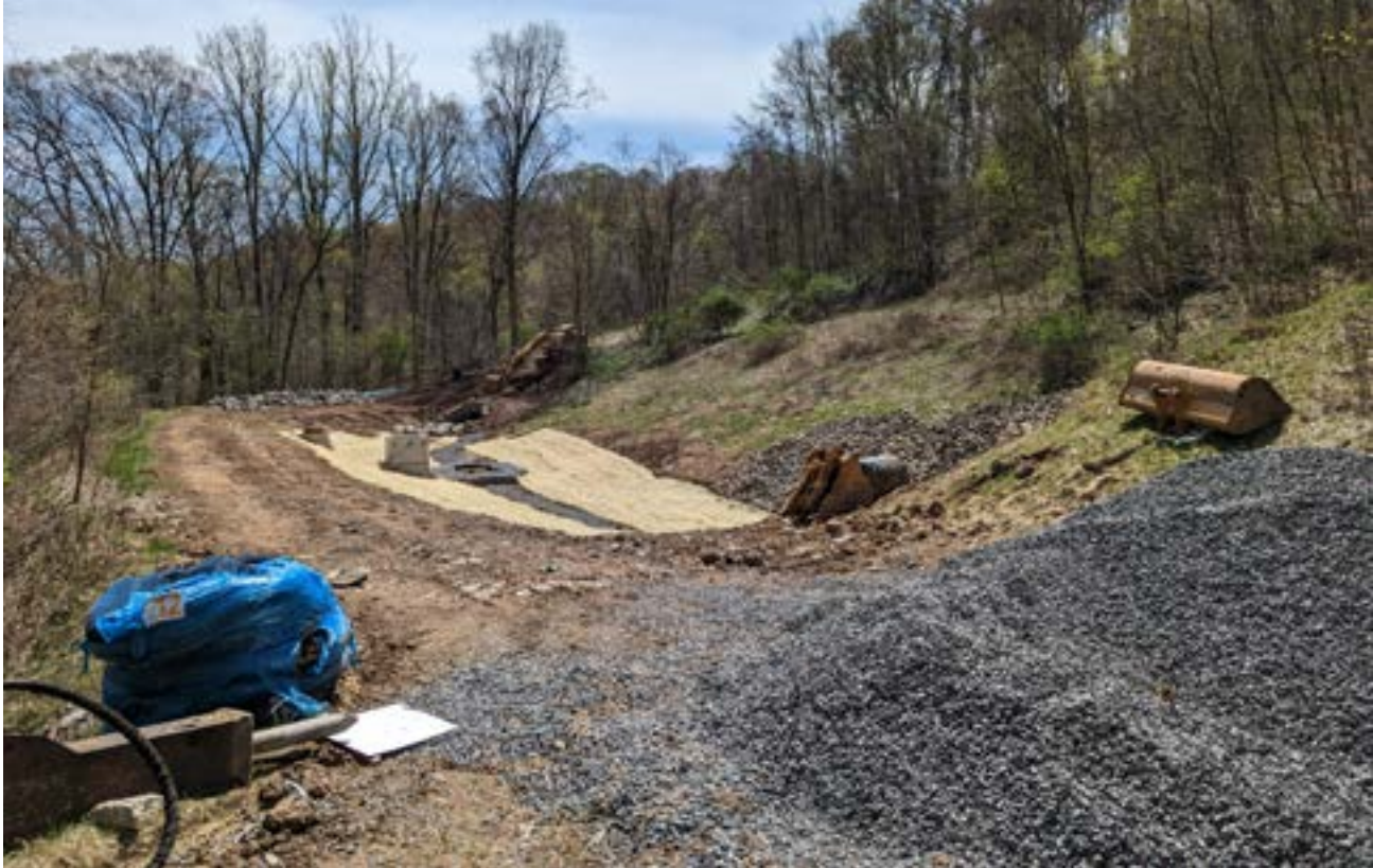
A Stormwater Detention Facility Along Mount Nebo Road in Ohio Township
