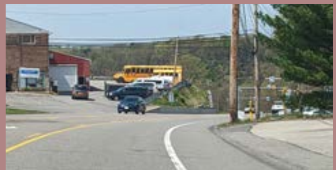
Roadway View of Existing Conditions Along Mt. Nebo Rd
