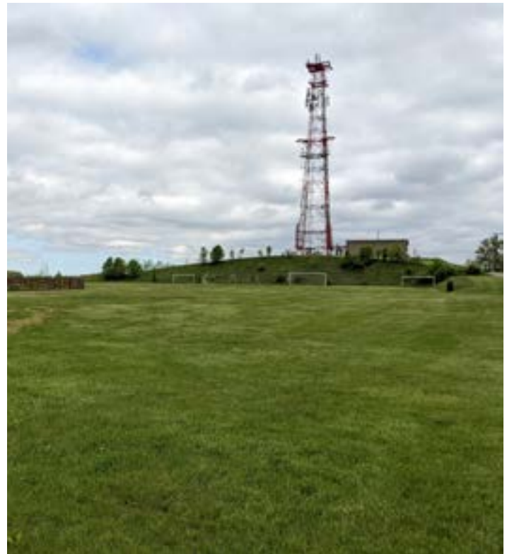
Cell Tower Overlooking Ohio Township Park
