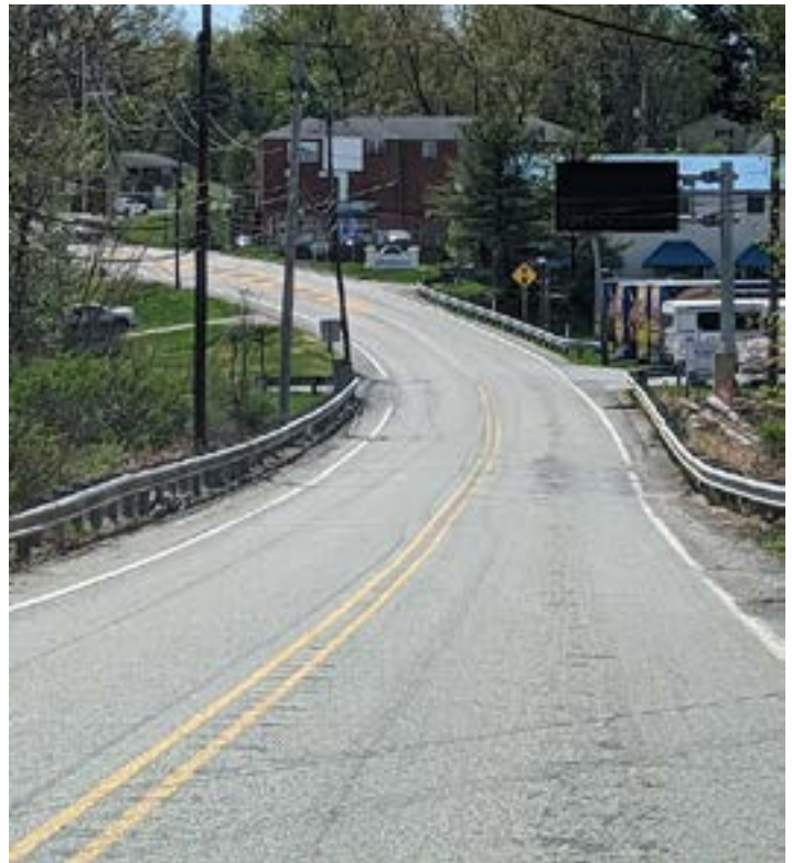
Nicholson Road in Ohio Township, Approaching Mount Nebo Road with Limited Shoulder
