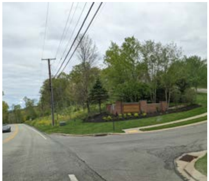
Entrance to Castletown Neighborhood in Franklin Park, Showing Internal Sidewalks without External Connection
