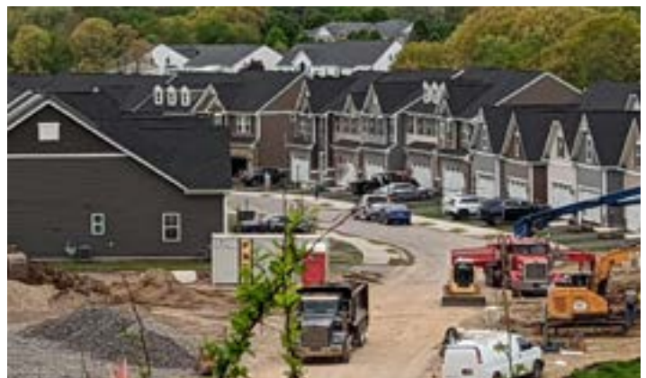
Sewickley Crossing Development Under Construction
