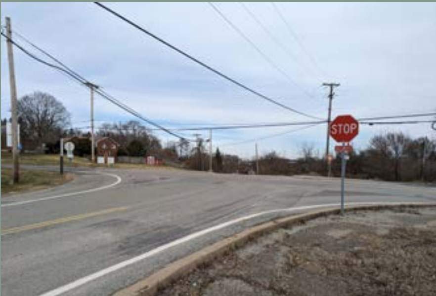
Roadway View of Existing Conditions from Rochester Road
