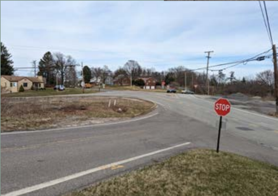
Roadway View of Existing Conditions
