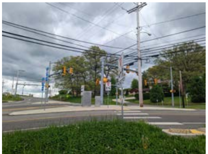
Nicholson Road and Mount Nebo Road Roadway
